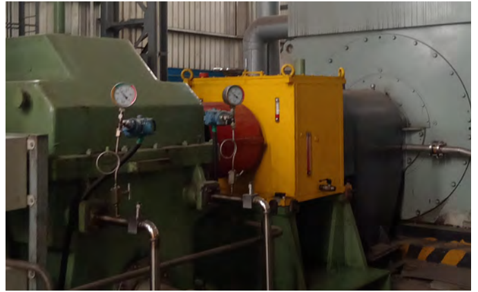
Housing Freewheel FH 60000 in fan drive
