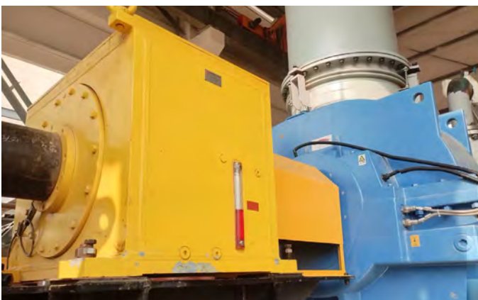
Housing Freewheel FH 42000 in circulating pump
